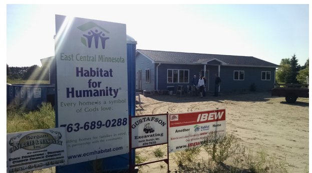
A new home under construction by East Central Habitat for Humanity
